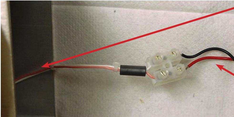
Remove end cap on right side of pump panel to expose wires
